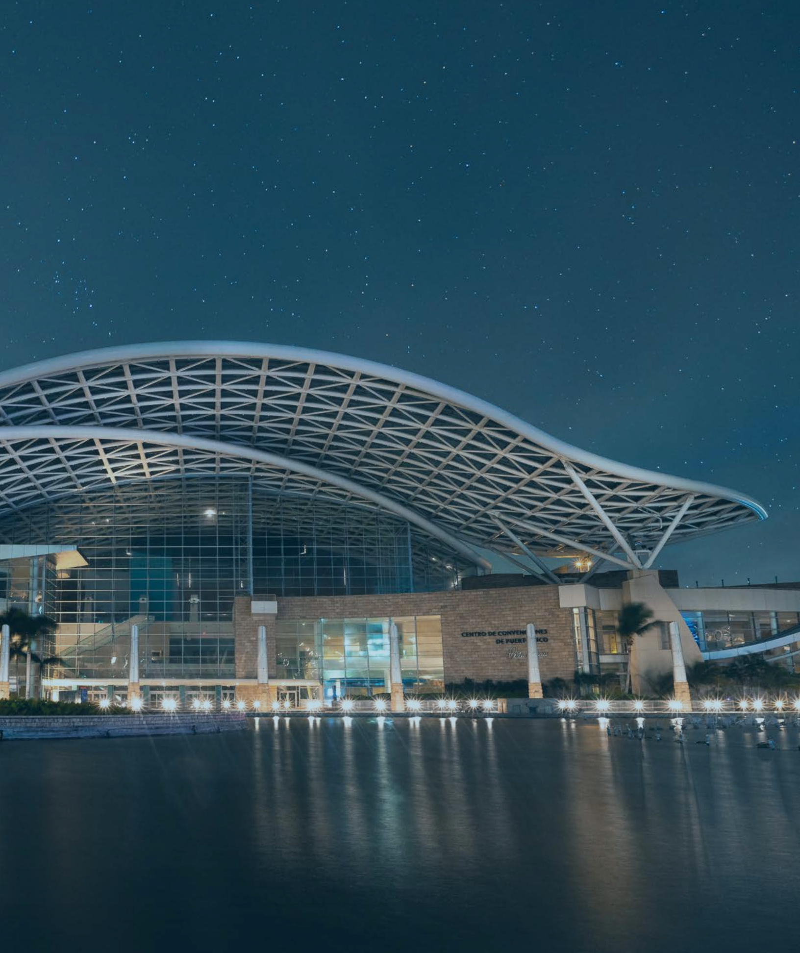
PUERTO RICO CONVENTION CENTER SAN JUAN, PUERTO RICO
